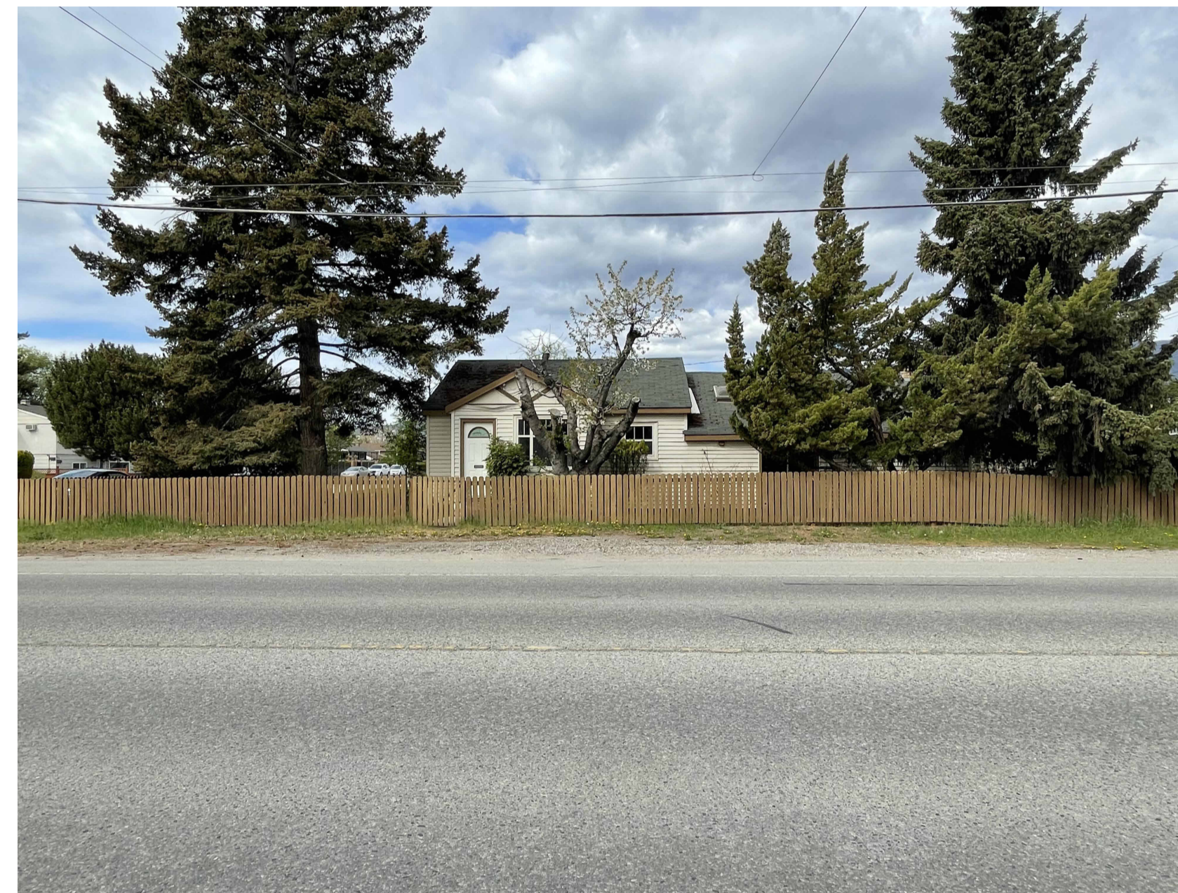
2. VIEW FROM RICHTER STREET FACING THE SITE
